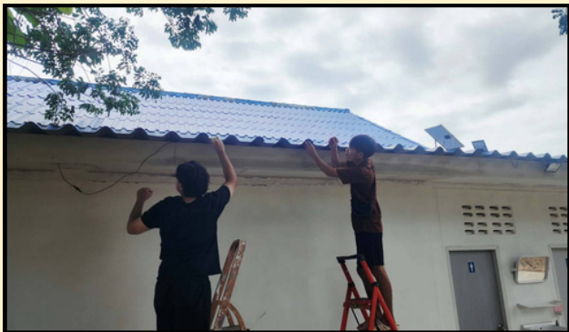
We added new solar lights along the walkway to improve lighting and safety.
