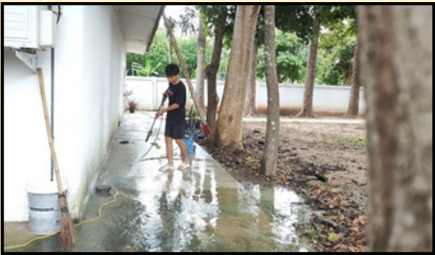
We power-washed the moldy walkway to make it safer and prevent slips and falls.
